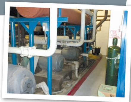
→ A clean compressor room allows leaks to be easily identified.
