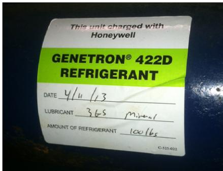
→ This is an example of a system that was converted from R-22 to Genetron 422D.
